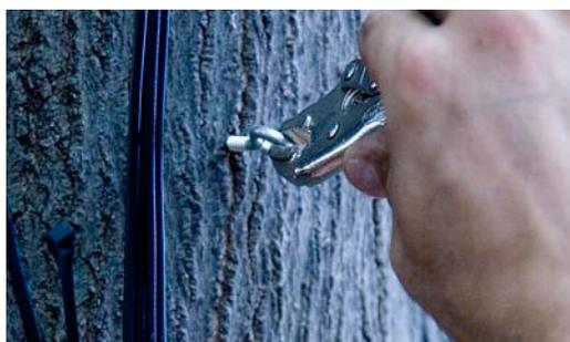
Step 1. Pre-drill hole then secure stainless steel screw eyebolt. Leave about 1" thread exposed.
