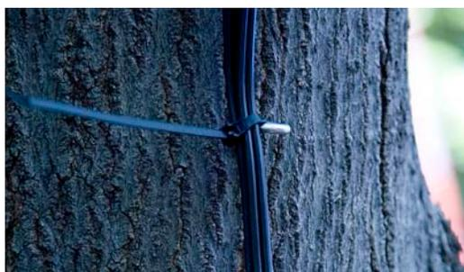
Step 3. Close cable tie loosely to allow for movement of cable through tie. Trim excess cable tie.
