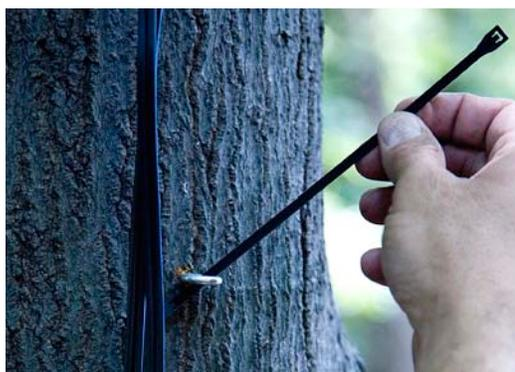
Step 2. Thread cable tie through eyebolt and around wire(s).
