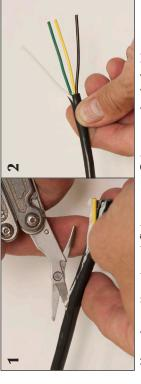
lead wire. Use small scissors or knife to strip away wire jacket. Use wire cutters to cut fixture
