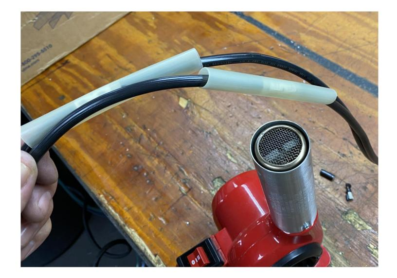
Starting at the center of the splice turn the wire to evenly heat the heat shrink and work your way to the ends. This helps remove any trapped air and moisture.
