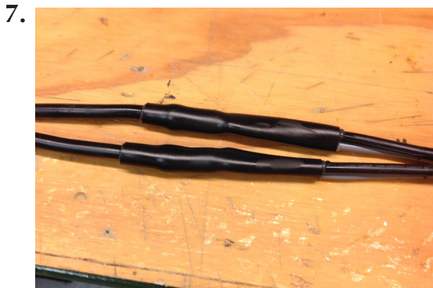
Completed Direct-Burial Heat Shrink and Butt Crimp Wire Splice Connection.
