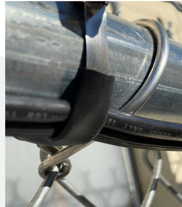
Close View of Sleeve Placed Over Wire
