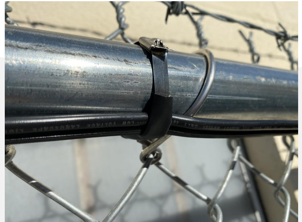
Finished Cable Tie Connection
